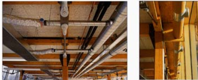
Figure 7: independence of subsystems in the “XX” building
